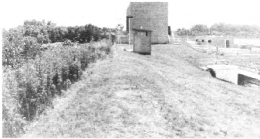
Figure 6. Dye injection shed and weather station
